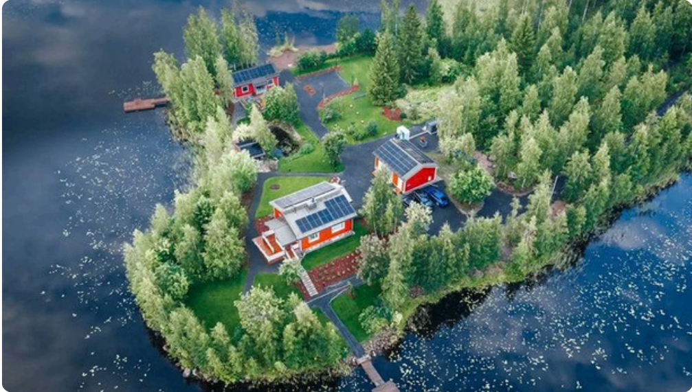
Pure Hydrogen Fuel Cell and Air-to-Water Heat Pump System
