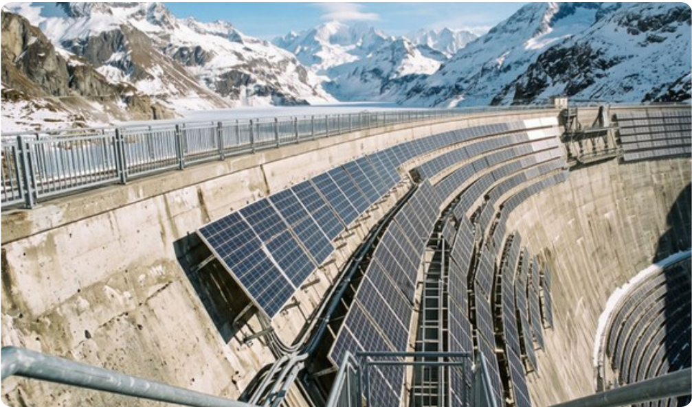
5,000 solar panels on a dam wall 8,000 feet up
